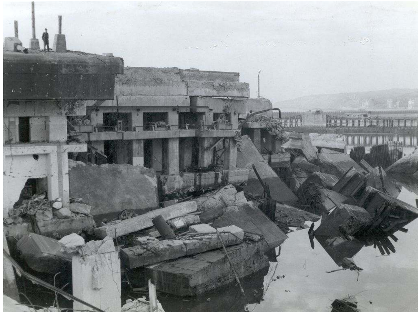
Damage to the E Boat Pens at Boulogne after the attacks of 15 June 1944
