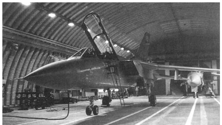
Fig 5-1 Physical protection - inside a hardened aircraft shelter (HAS)
